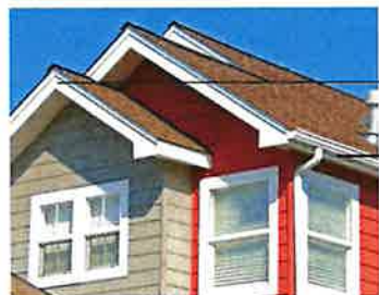
Rake Overhanging Eave Overhanging
