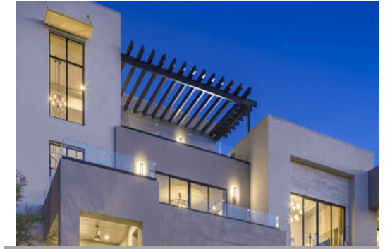
TRELLIS SHADE STRUCTURE
